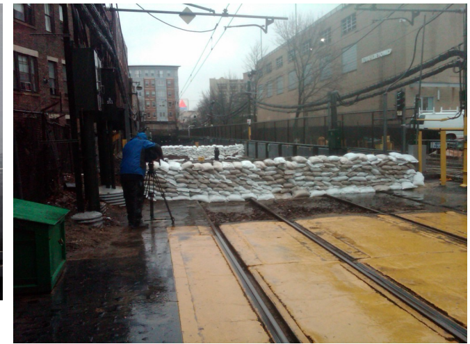
Figure 5: The MBTA places dams at the Fenway portal in Boston, MA due flooding of over 15 feet from the nearby Muddy River (MassDOT, 2010).
