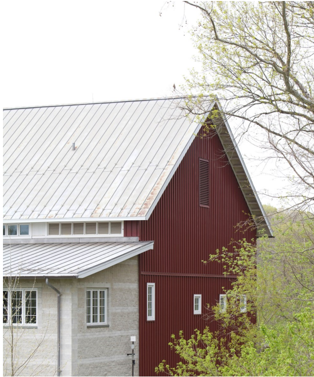
Figure 23: A white roof atop a building. White roofs absorb less heat than darker colors (Hagerty, n.d.).
