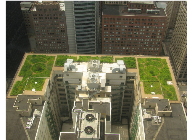
Figure 22: A green roof atop the 10-story Chicago City Hall. Roofs like these can provide greenery in environments that otherwise have little space for them (TonyTheTiger, 2008).
